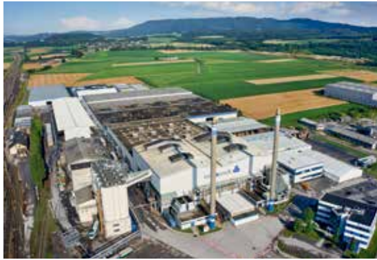
Pöchlarn Plant, Austria
